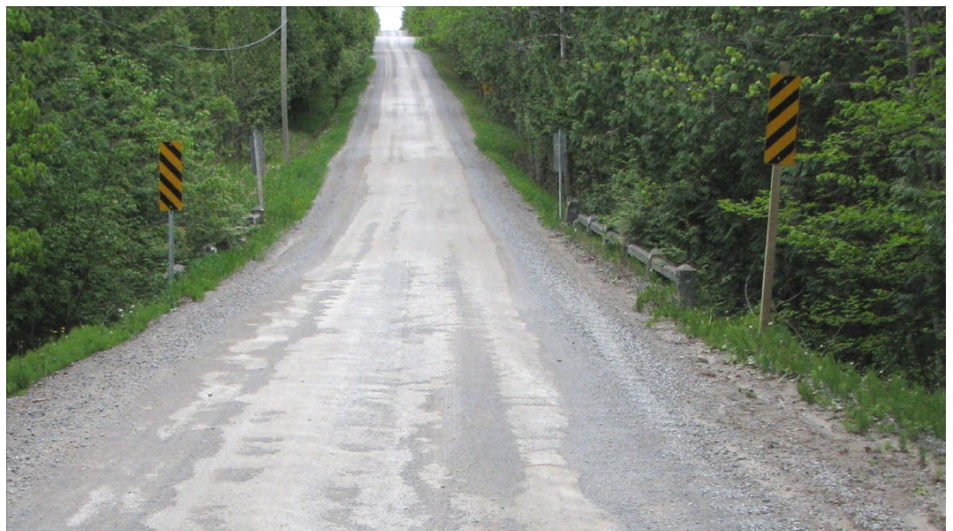
Buried bridge in the GTA, T-beam with open railings.
