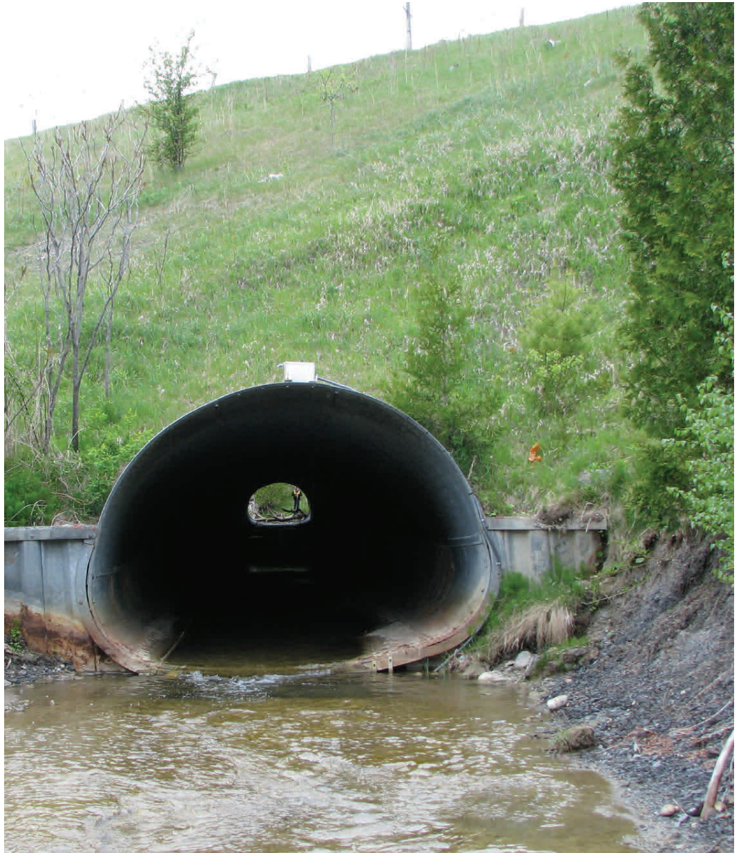
Perforated 1980's vintage 64 m long CSP with 10 m cover will need $1M replacement by 2025
