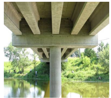
Prestressed girder bridge in Prescott-Russell Counties.
